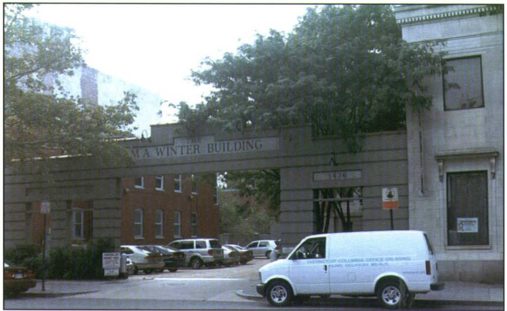
Figure 5 - The M. A. Winter Building today
